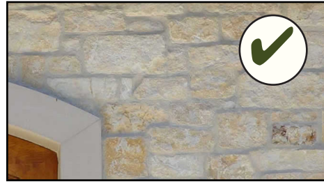
Rough stone laid in a random-ashlar pattern is appropriate for the Historic District.
